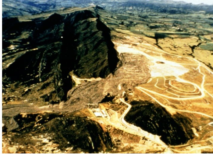
Figure 3: Photo of landfill slope failure in South America caused by excessive deep interior injection well pumping activity into light-weight lift compacted solid waste fill materials
