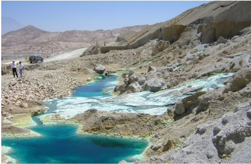
Figure 2: Photo of leach pad slope failure in South America caused by a combination of seismic activity, piping and saturated loose ore heap fill conditions in the downhill exterior slope
